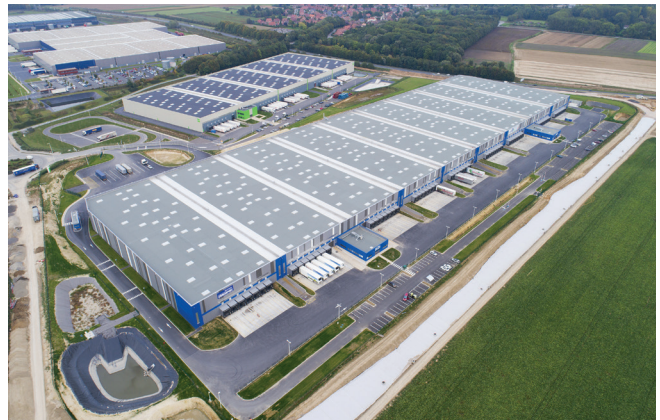
Lauwin-Planque Logistics Centre
